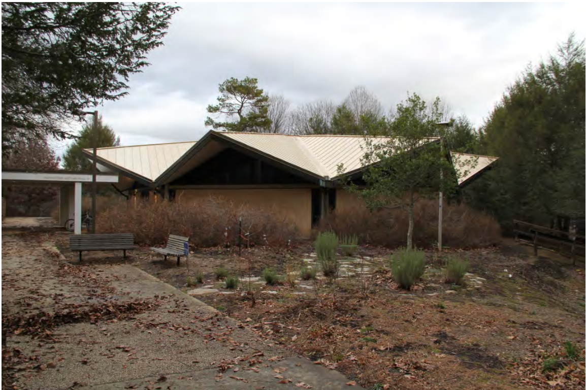
(#7) Humanities Lecture Hall (1966), oblique view to northeast
