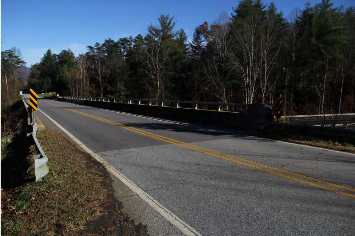
Bridge No. 367 on SR 1720 (Aiken Road) over US 19-23, view to east
