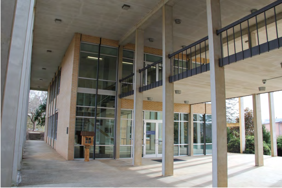
(#14) Phillips Hall (1961), view to south
