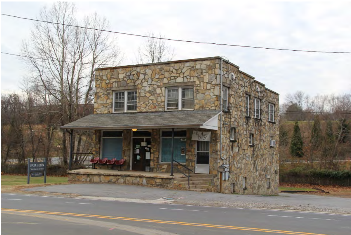
Commercial Building, 130 Weaverville Road, oblique view to southwest
