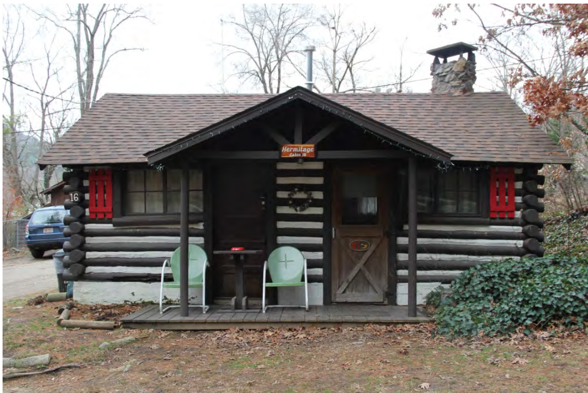
Hermitage, ca. 1935, façade, view to south
