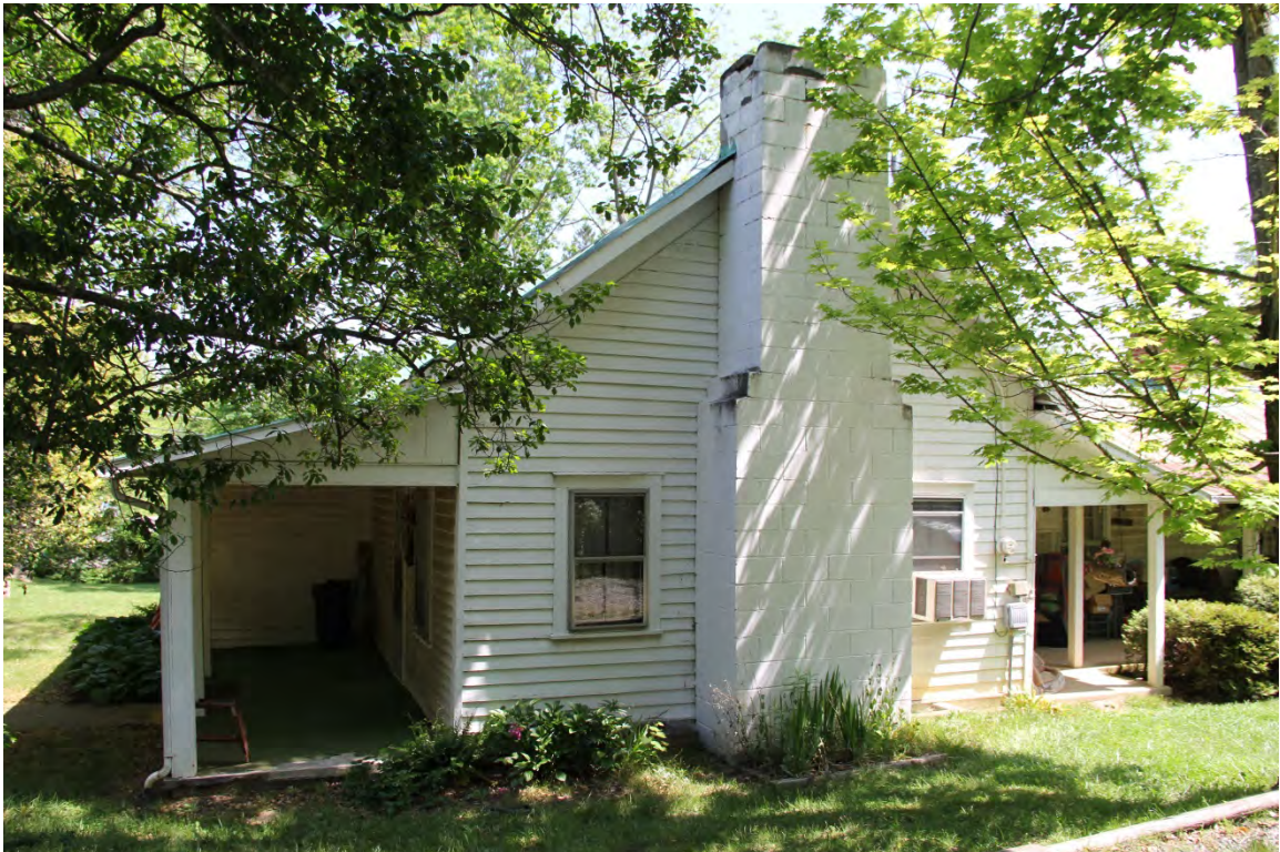
Mackey House, south elevation, view to north
