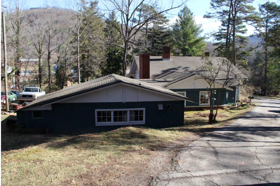
Office, rear wing, view to east
