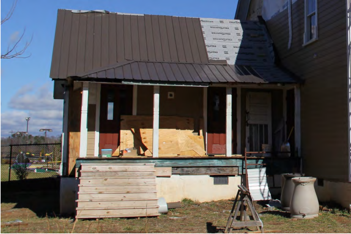
Baird House, rear ell, view to north
