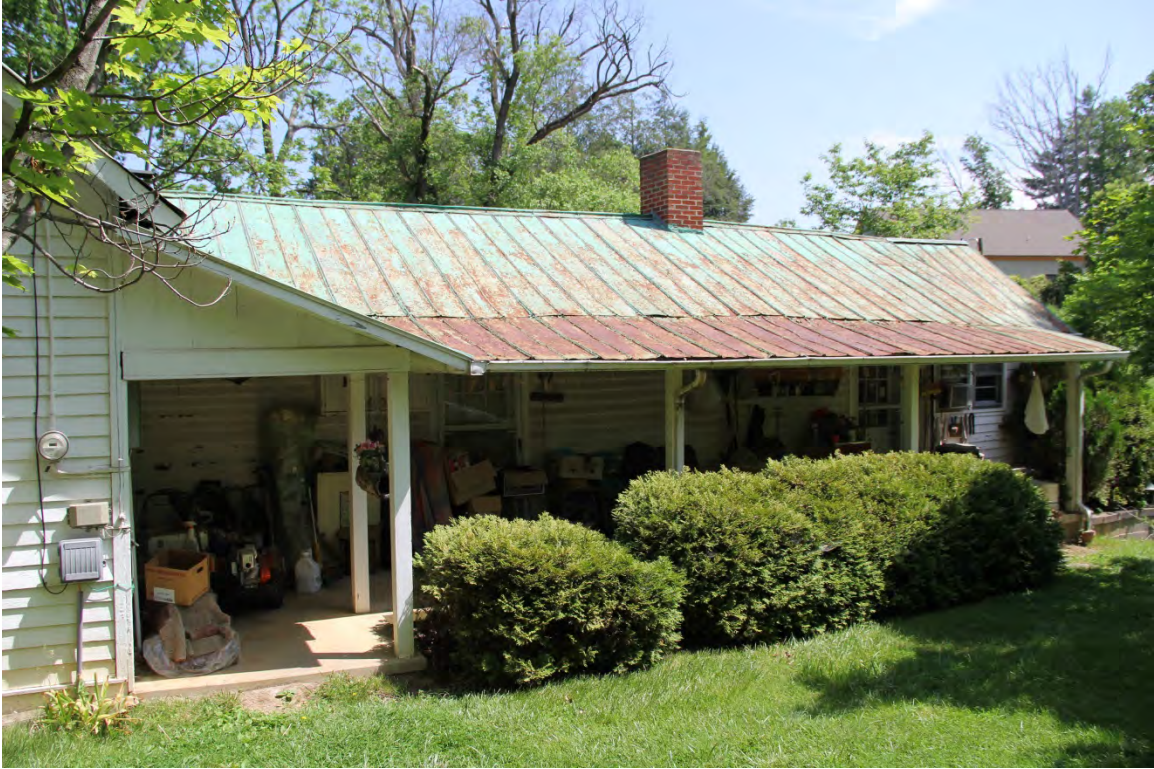
Mackey House, south elevation of rear ell, view to north
