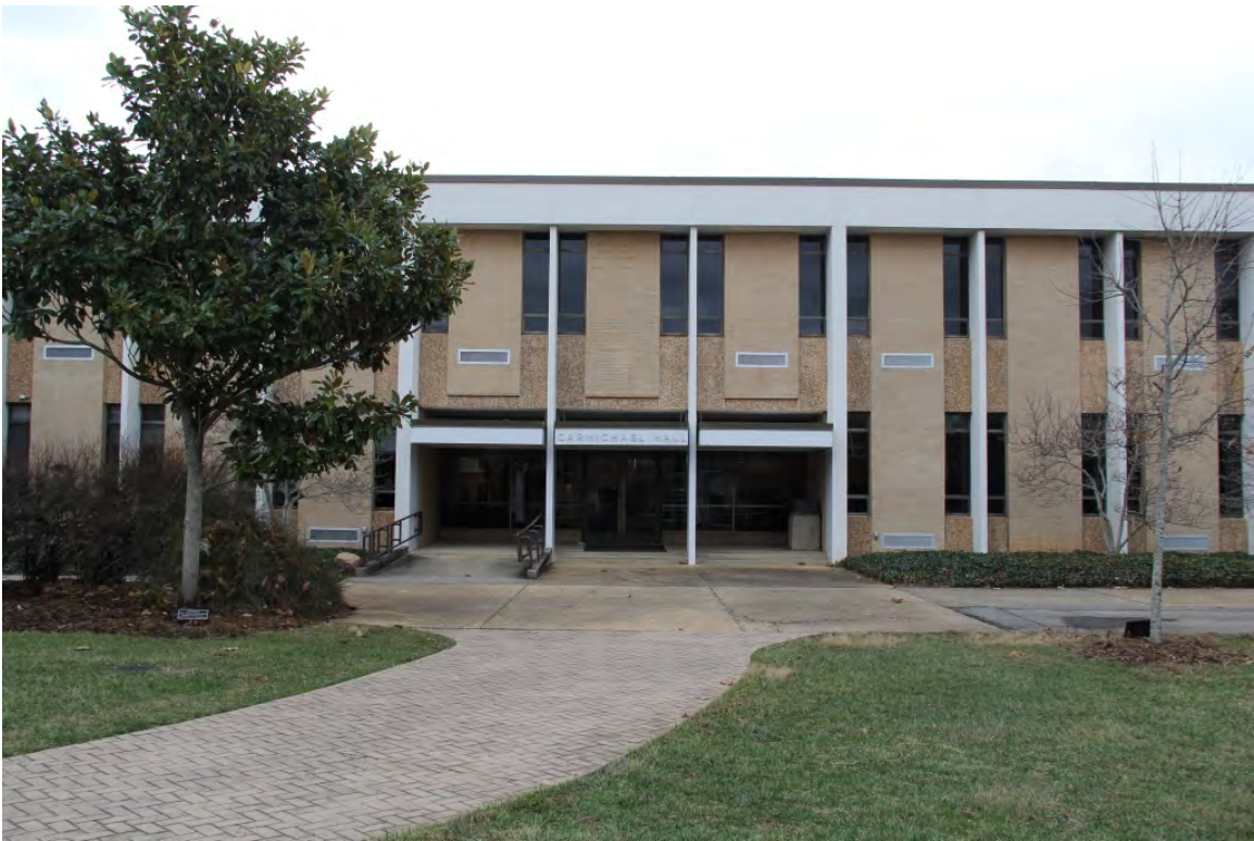
(#4) Carmichael Hall (1966), façade, view to southeast
