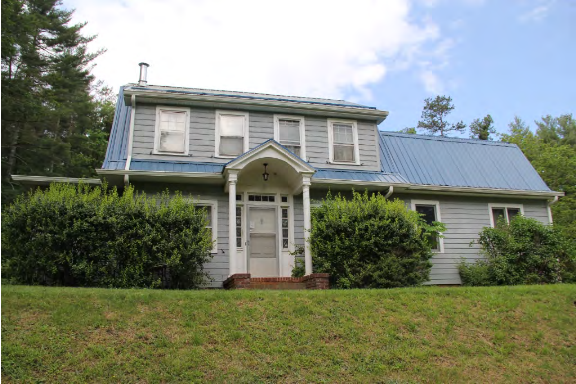
Ward House, façade, view to southwest
