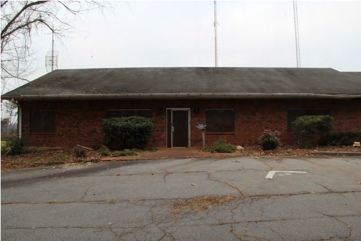
WISE Office, façade, view to west
