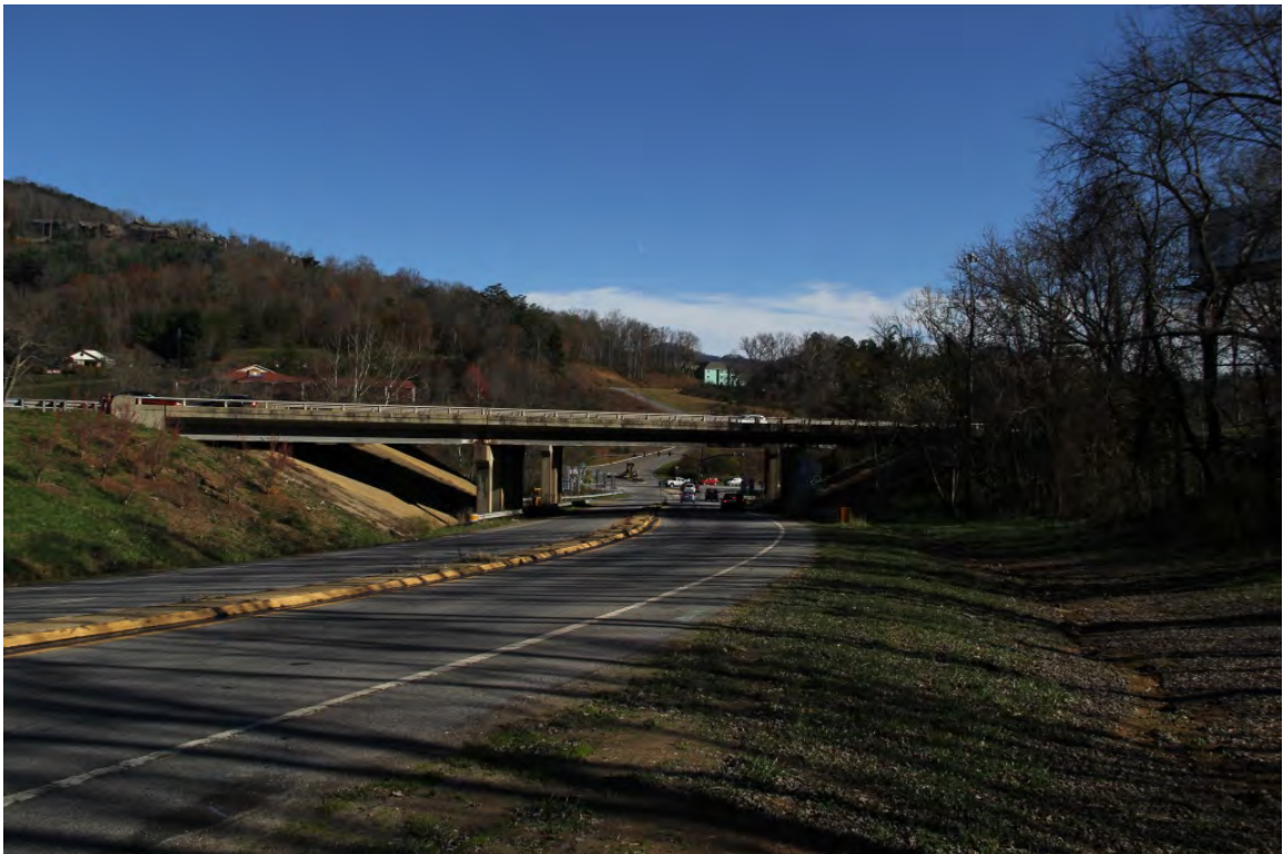
US 25 (Weaverville Road) interchange, Exit 23, view to southeast
