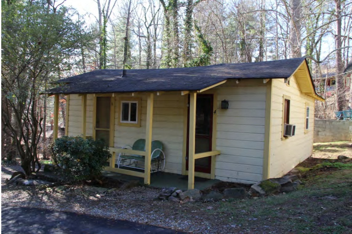
Sitnwhittle, façade, view to southwest
