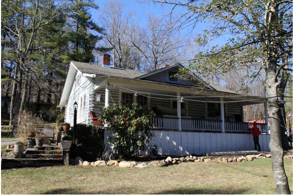
Office (The Homestead), façade, view to northwest
