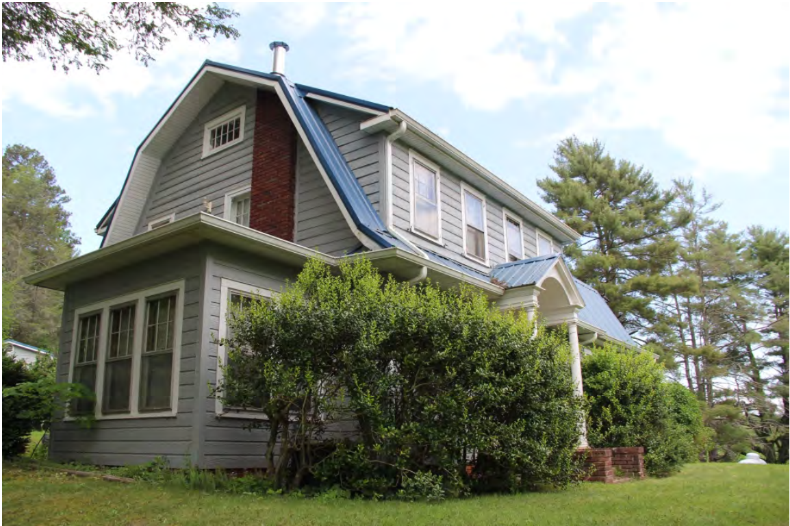
Ward House, oblique front view to north
