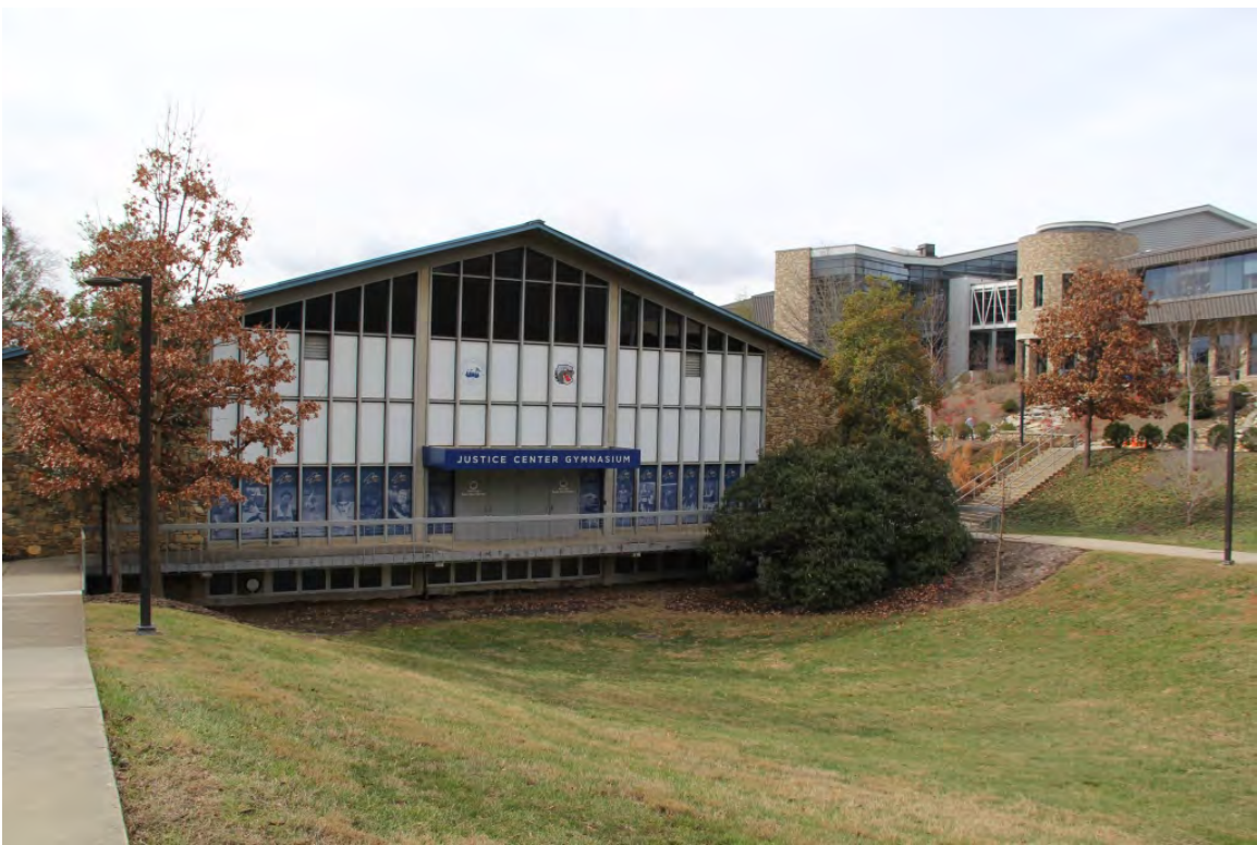
(#8) Justice Center Gymnasium (1963), view to west
