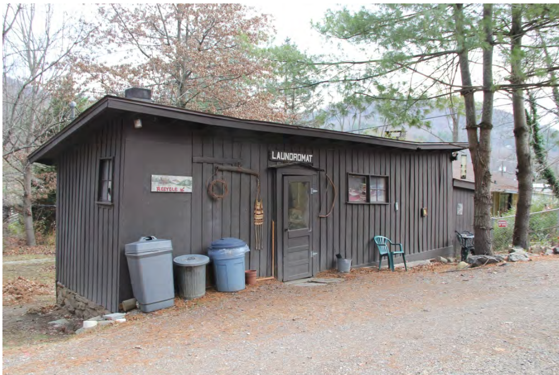
Laundry, ca. 1935, oblique front view to southeast
