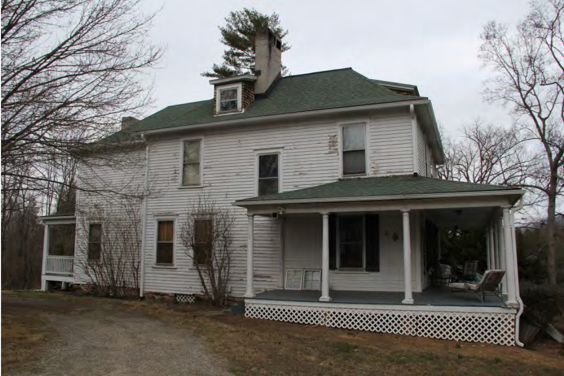
McPherson House, south elevation, view to north
