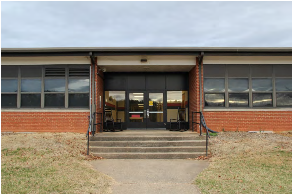
North classroom wing, entrance, view to east
