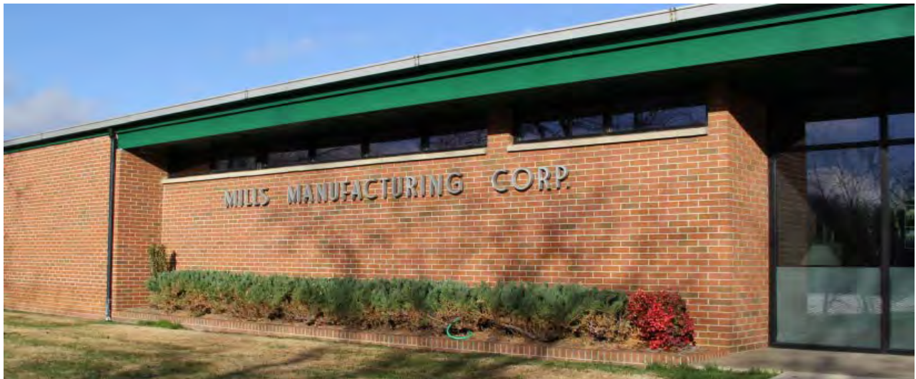
Mills Manufacturing Corporation, 25 Mills Road, oblique front view to northwest
