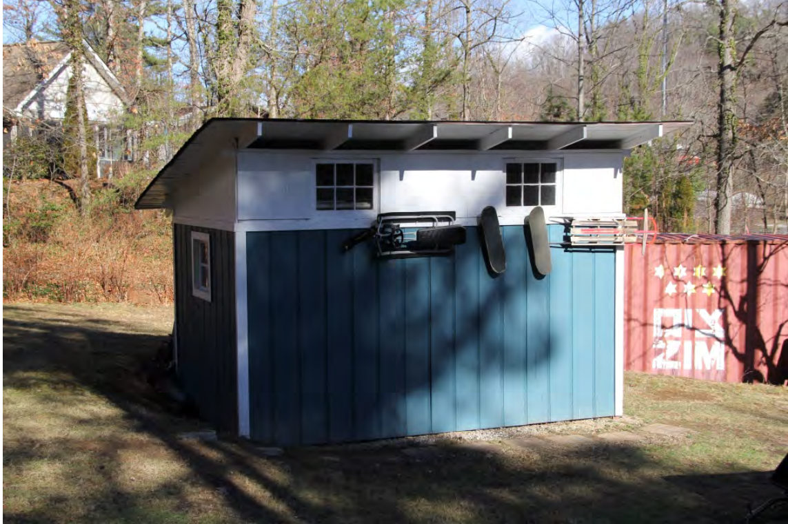
Storage building, view to southeast
