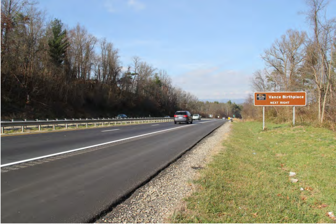
View to north along US 19-23, north of Heavner Road (Old Marshall Highway) overpass
