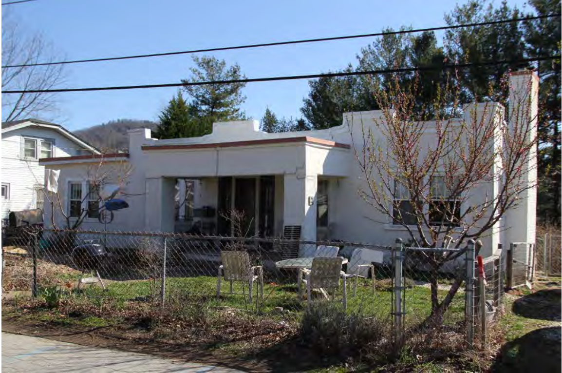
Lyday House, oblique view to northeast
