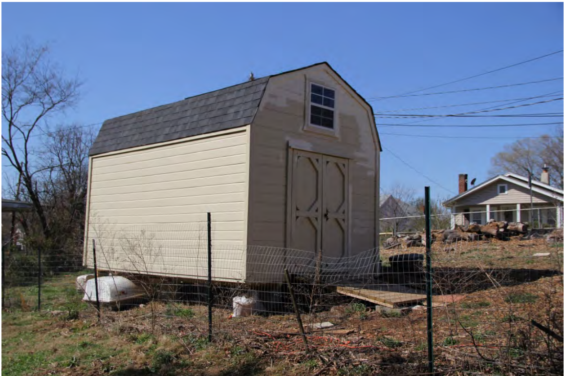
Shed, view to southwest
