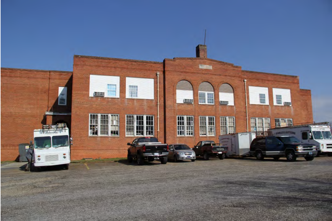
Façade, view to northwest
