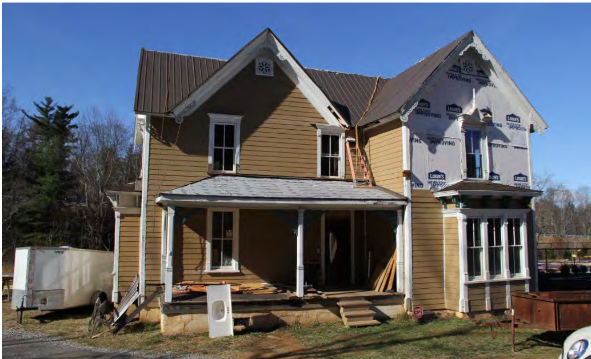
Zebulon H. Baird House, 446 Weaverville Road, façade, view to west
