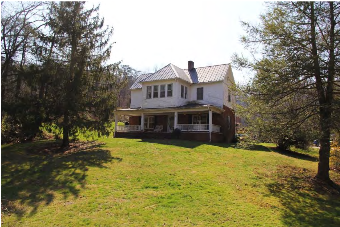
Blackstock-McElroy House, 66 Boles Cove Road, view to southeast
