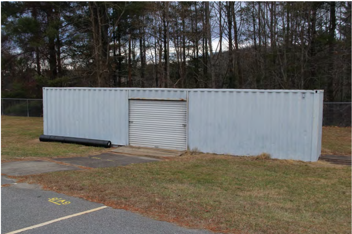
Storage building, facade, view to east
