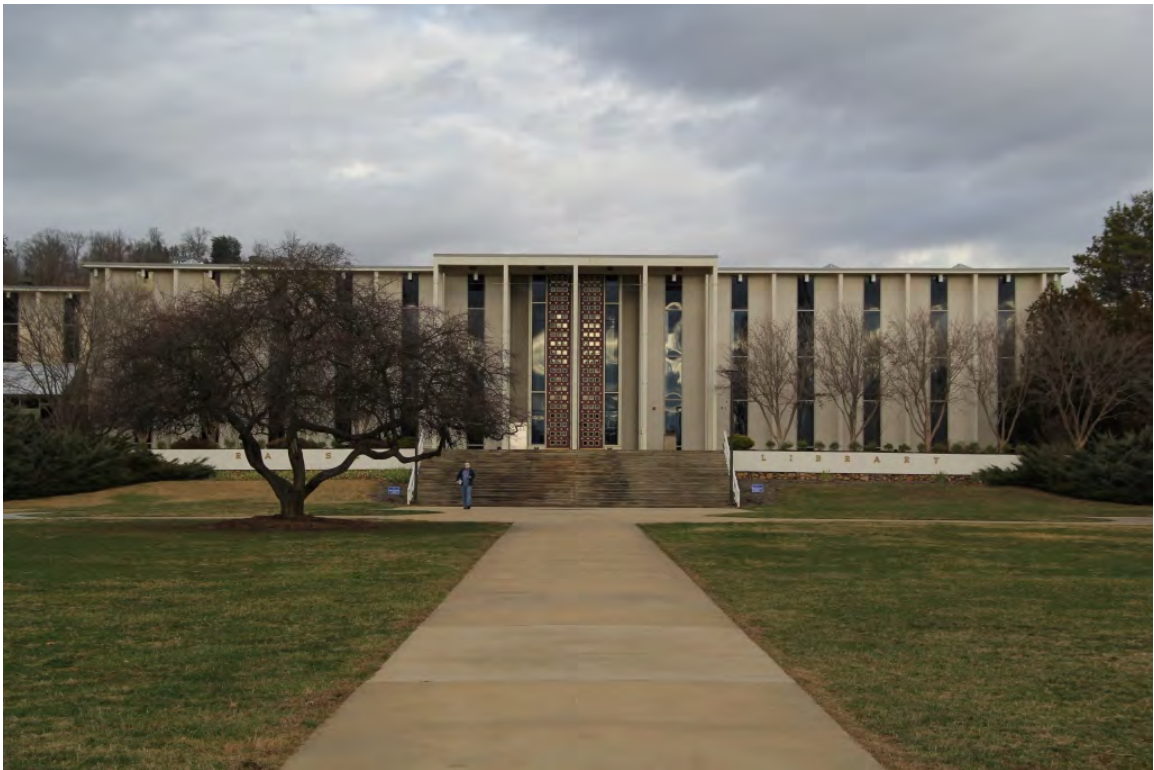
(#15) D. H. Ramsey Library (1965, enlarged 1990), façade, view to northeast
