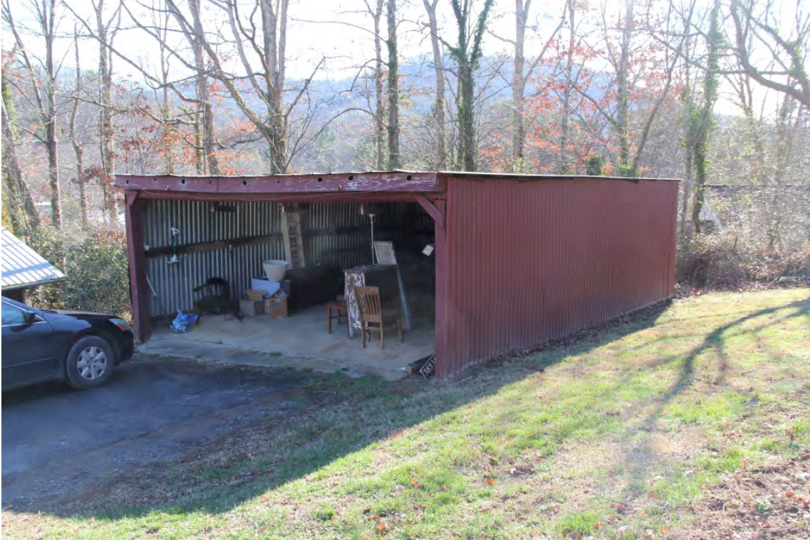
Garage, view to southeast
