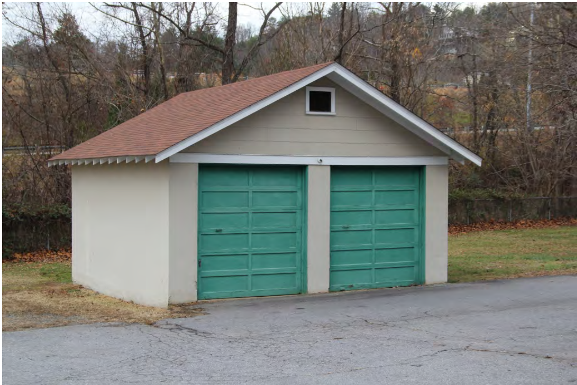
Garage, 132 Weaverville Road, view to west
