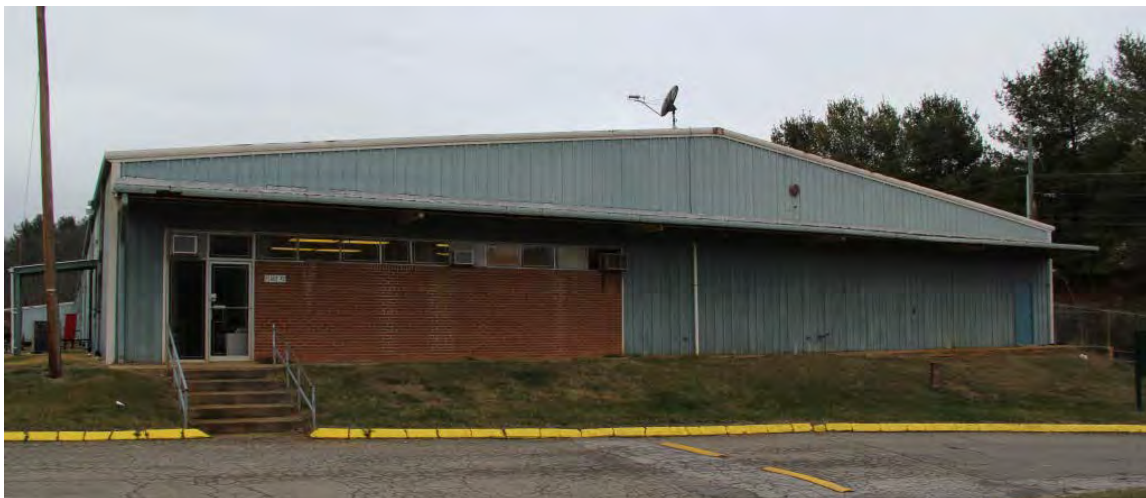
Mills Manufacturing, Plant No. 2 (ca. 1970), façade, view to west
