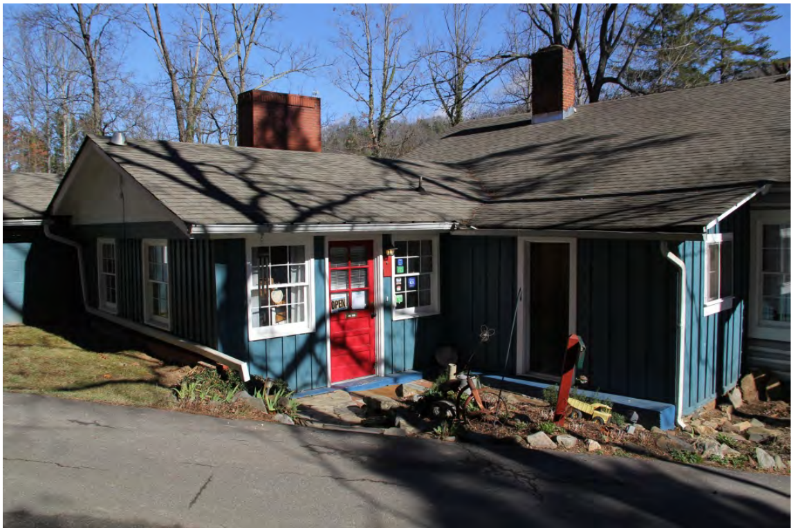
Office, oblique rear view to northeast
