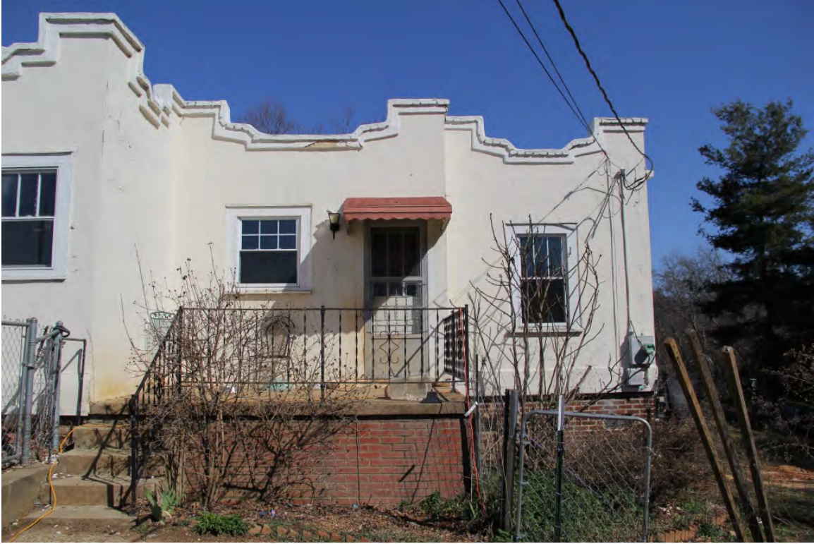
Lyday House, south elevation, view to north
