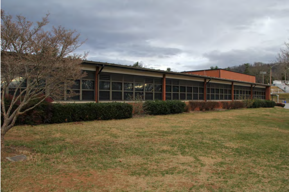
South classroom wing, view to southeast
