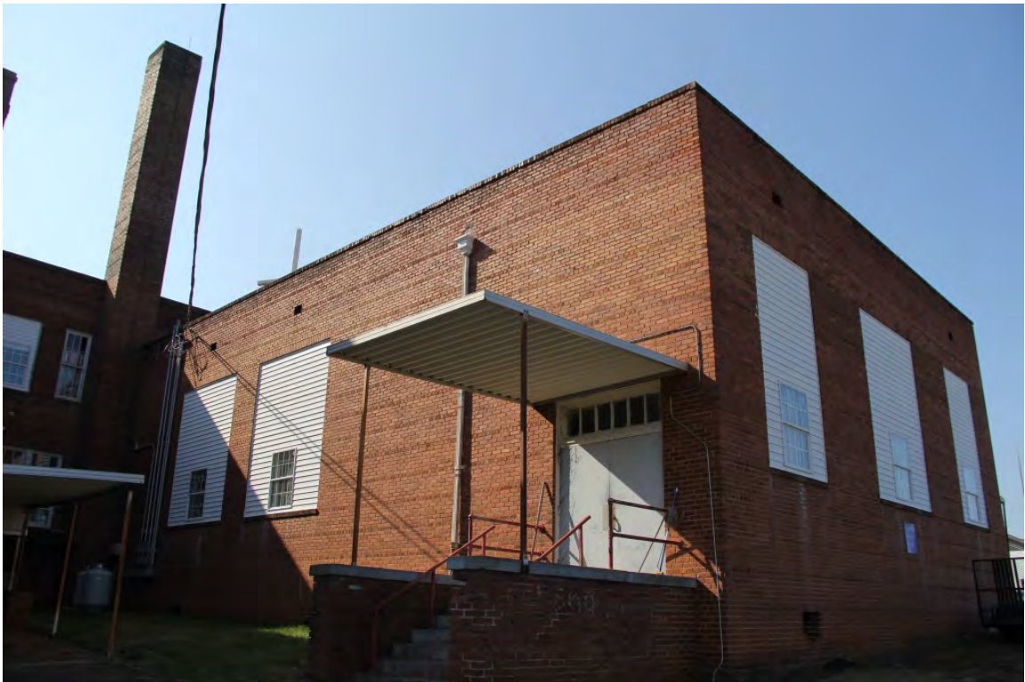
Auditorium wing, north side elevation, view to south
