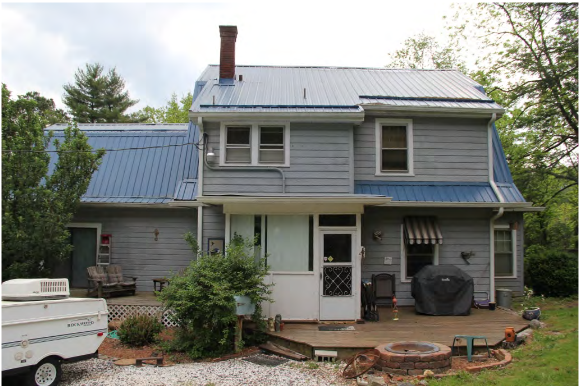
Ward House, rear elevation, view to east
