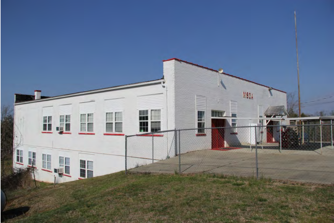
Cafeteria, oblique view to southwest
