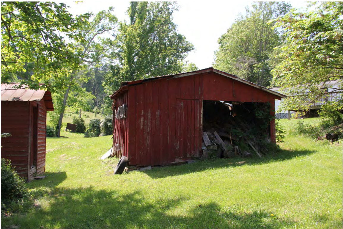
Tractor shed, façade, view to southeast; mobile home visible in background
