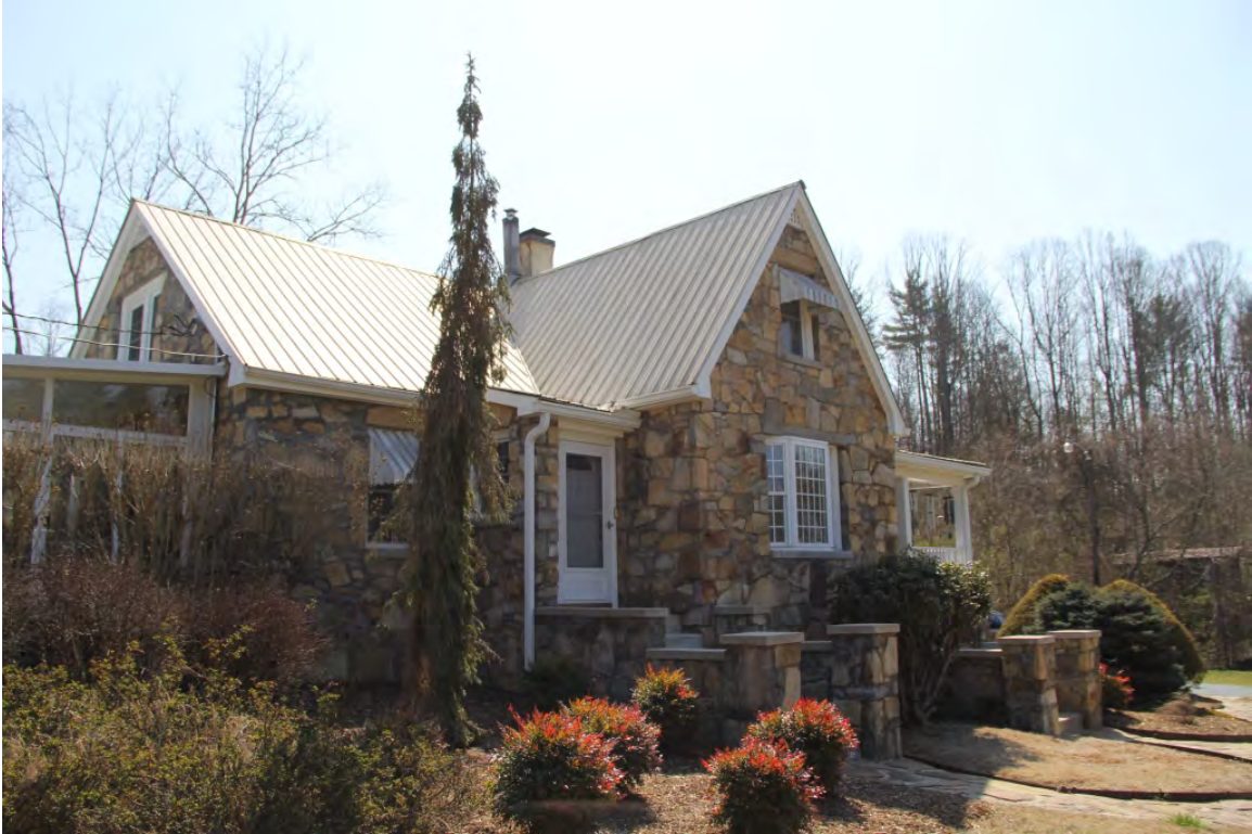
Banks House, oblique view to southeast
