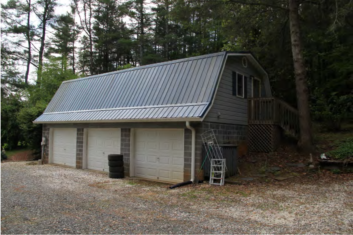
Garage/apartment, oblique front view to southeast
