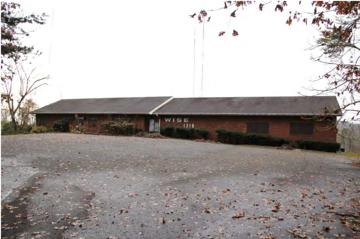
WISE Office, 27 Relic Lane, façade, view to west
