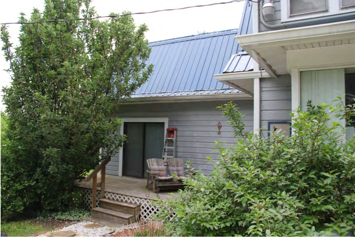
Ward House, north wing, rear elevation, view to northeast
