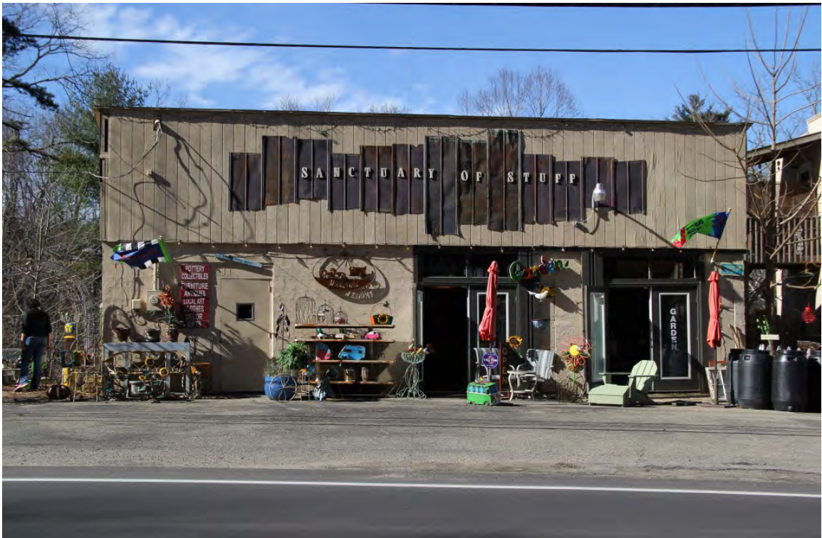
Service garage, façade, view to west
