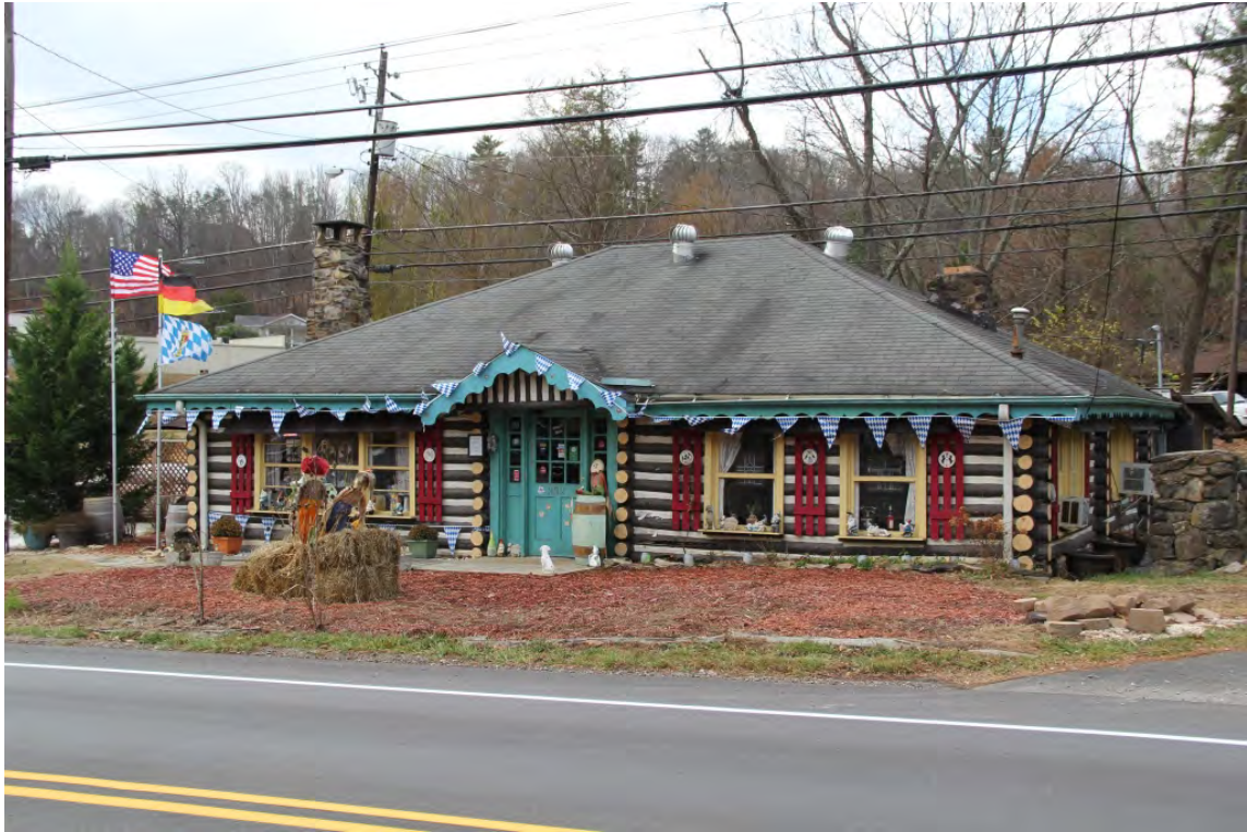
Dining Lodge, 332 Weaverville Road, 1937, view to southwest
