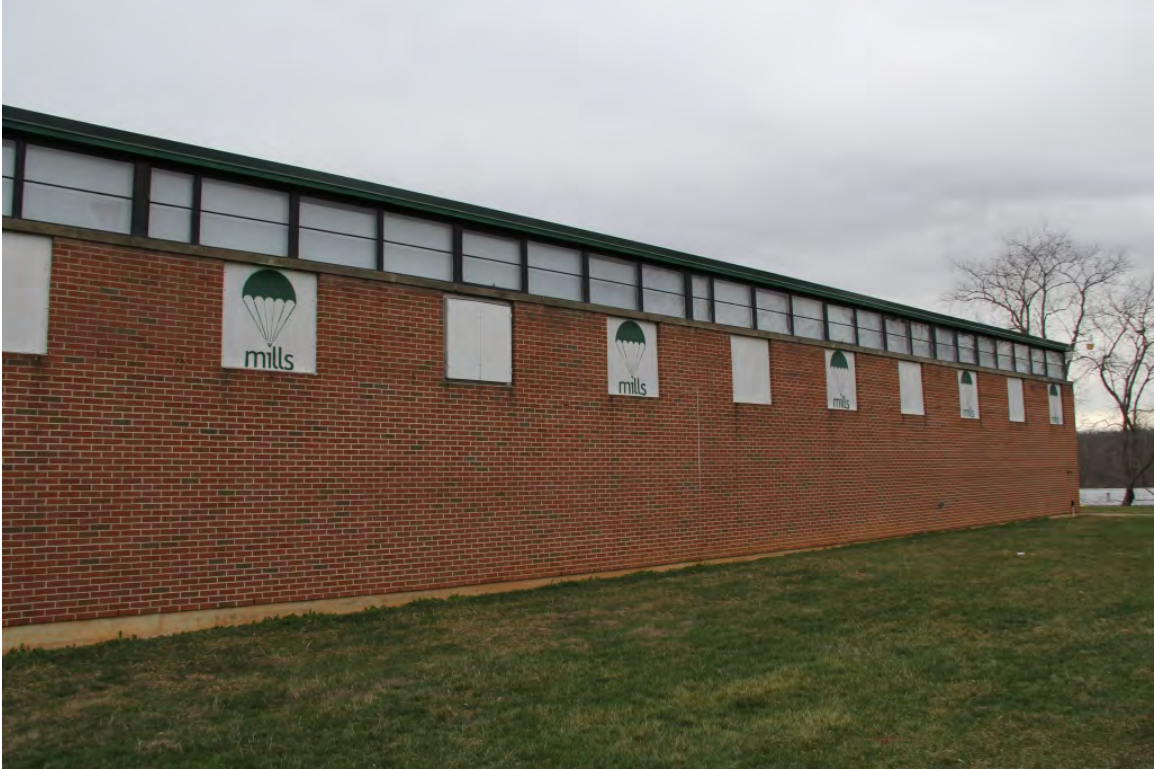
Mills Manufacturing, west elevation, oblique view to southeast
