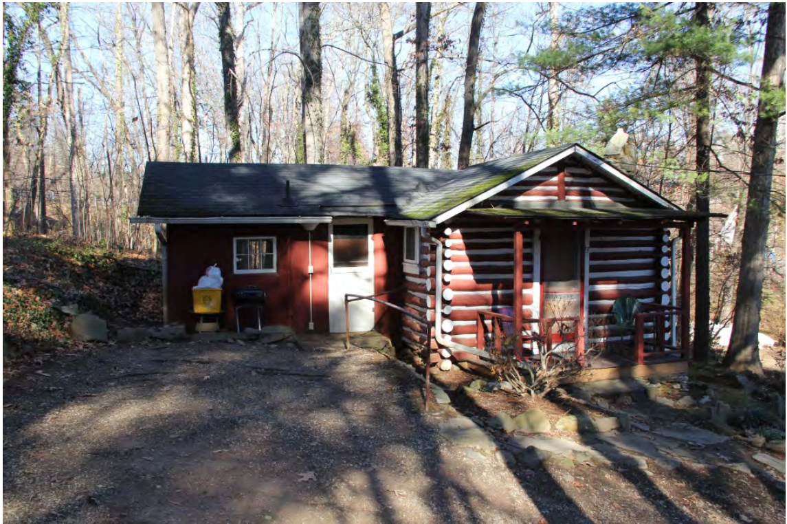
Havenden, façade, view to north
