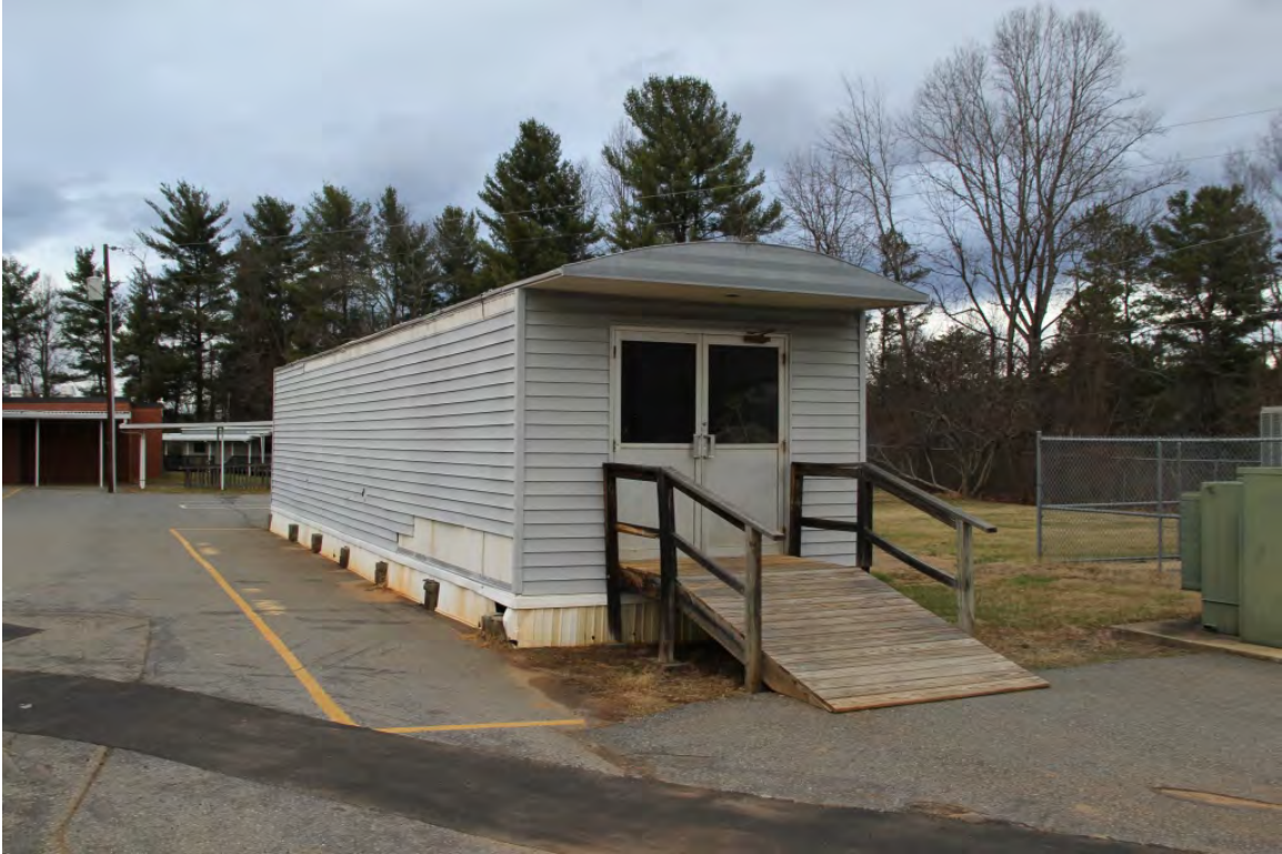
Storage trailer, view to north
