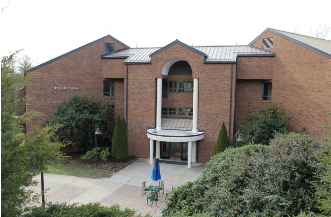
(#30) Mills Residence Hall (1987), façade, view to southwest
