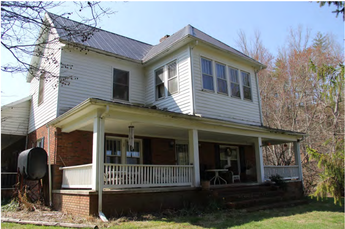
Blackstock-McElroy House, north side elevation, view to southwest
