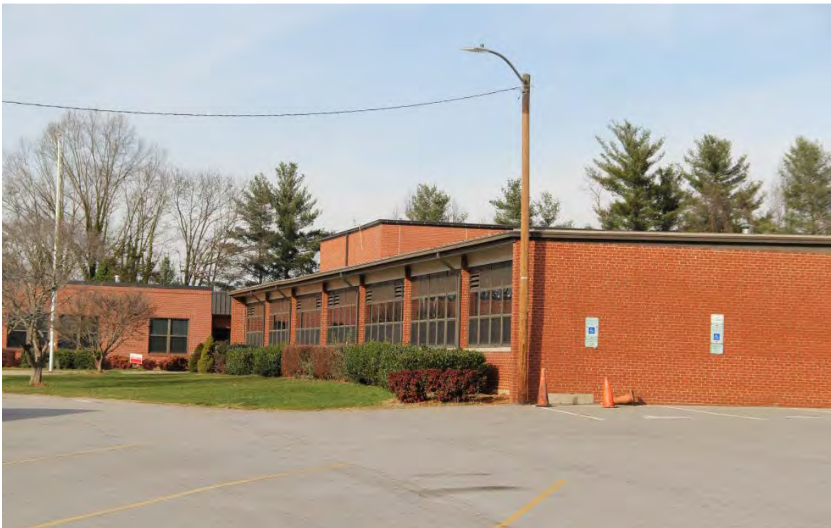
North Buncombe School, 51 N. Buncombe School Road, oblique front view to north
