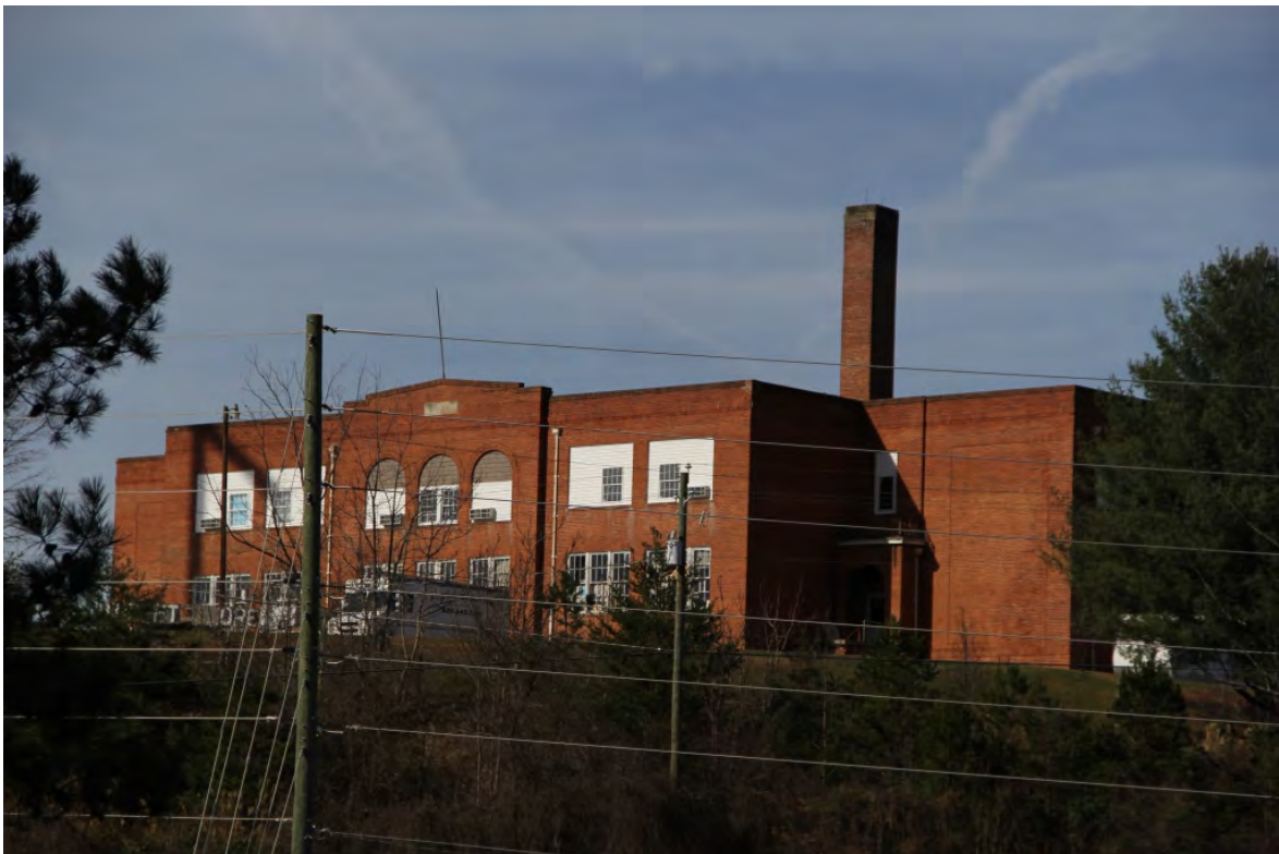
Flat Creek School, 20 Flat Creek School Road, view to west from US 19-23
