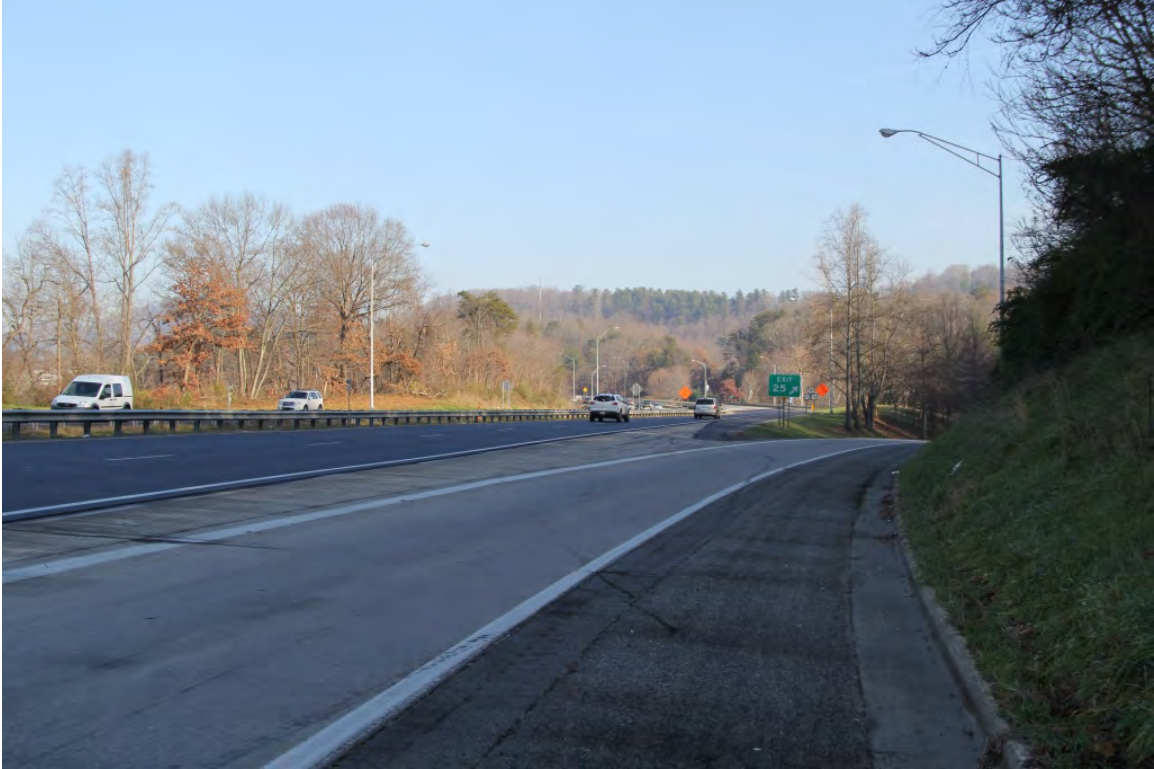
Project beginning, Exit 25, view to northeast along US 19-23
