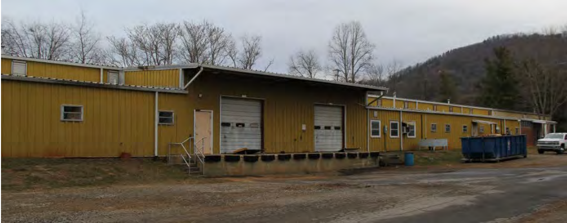
Mills Manufacturing, Plant No. 3 (1966), oblique front view to northeast
