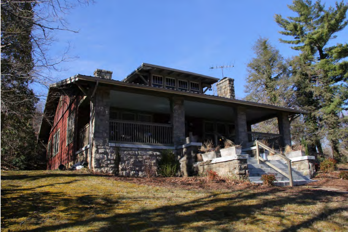
Sevier House, oblique view to northwest
