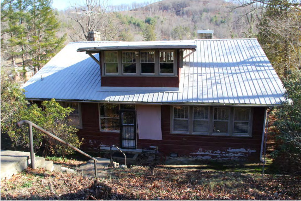
Sevier House, rear elevation, view to east
