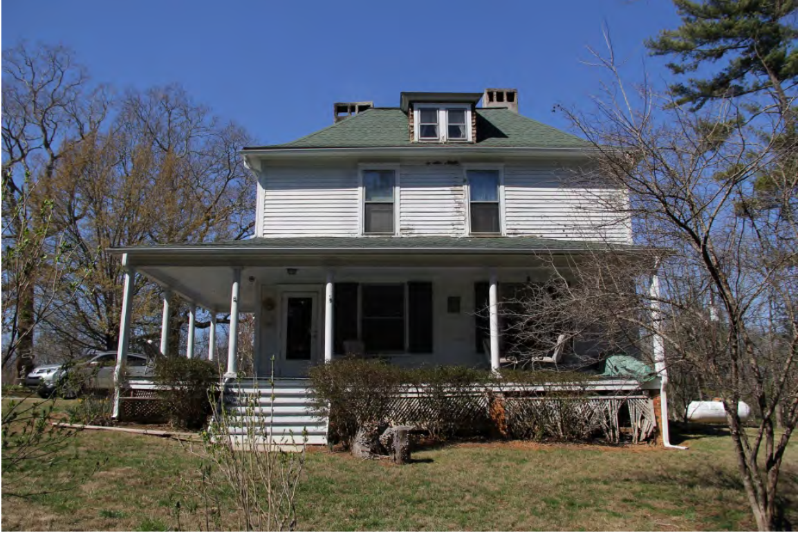
McPherson House, facade, view to west
