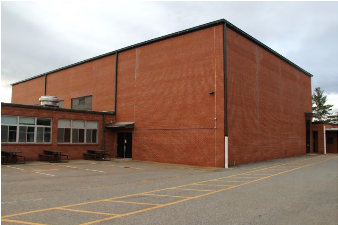
Auditorium, oblique rear view to northwest
