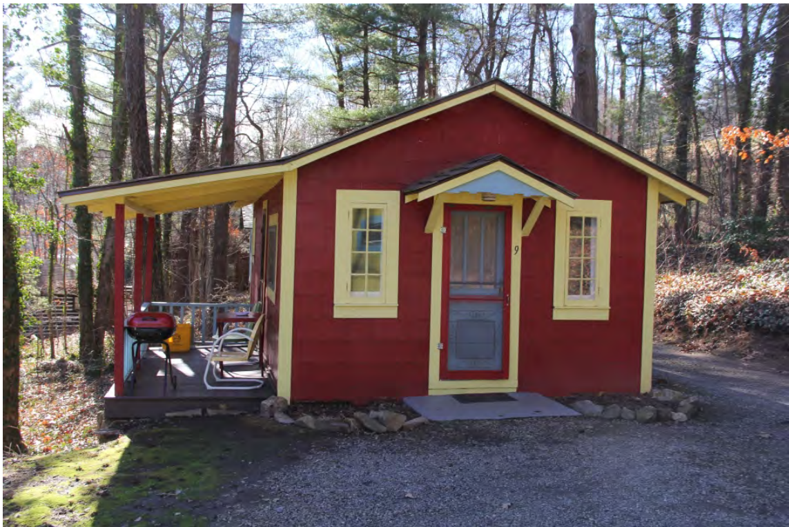
Overlook, oblique view to south
