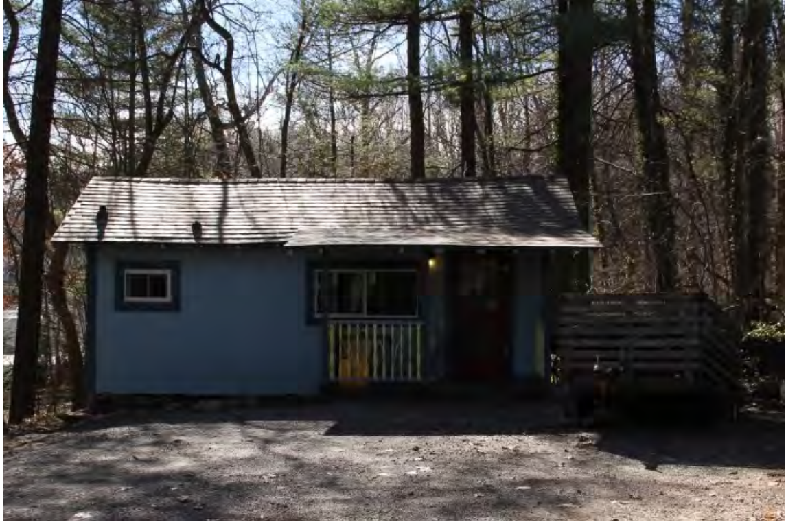
Dogwood, façade, view to south
