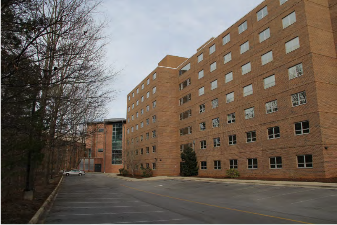
(#32) Founders Hall (1982), oblique view to northeast
