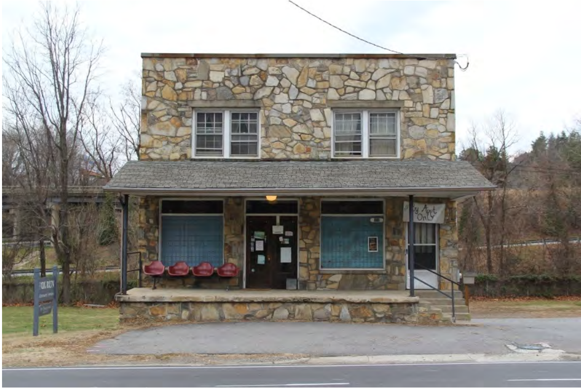
Commercial Building, façade, view to west
