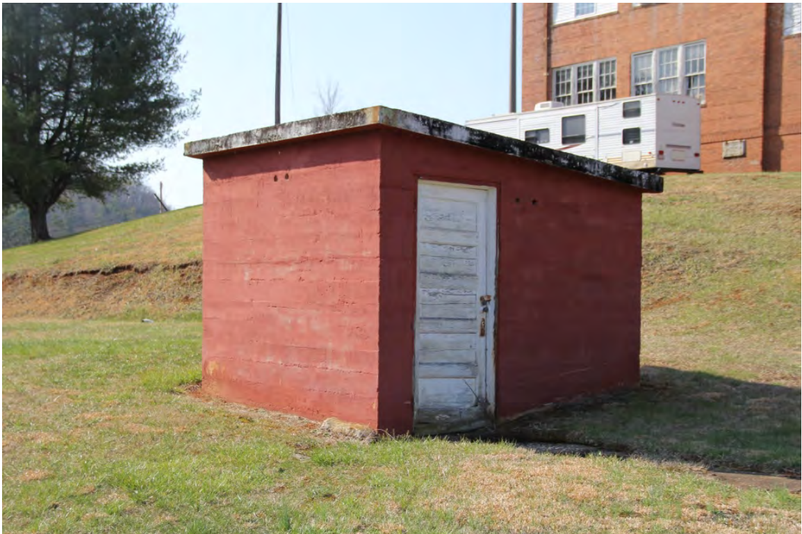
Pump house, view to south
