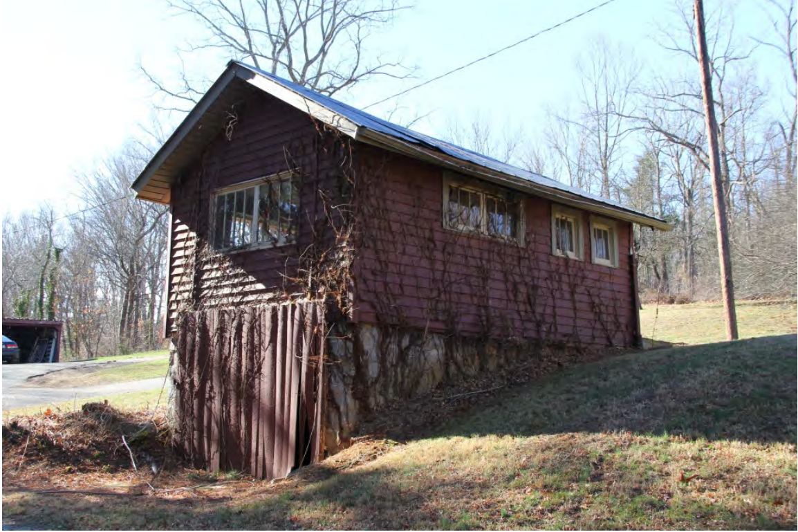
Outbuilding, oblique view to southwest
