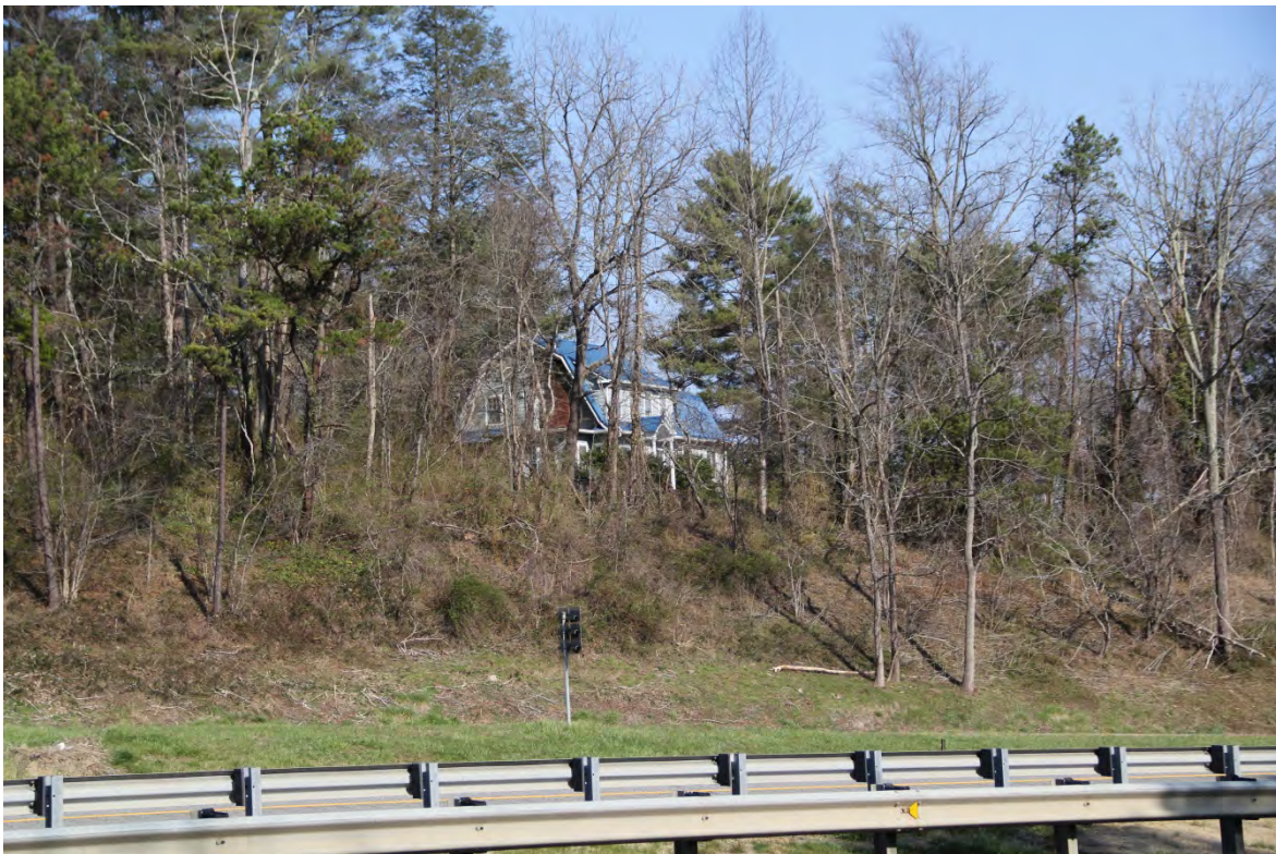
George and Inez Ward House, 75 Cole Road, oblique front view to west from US 19-23
