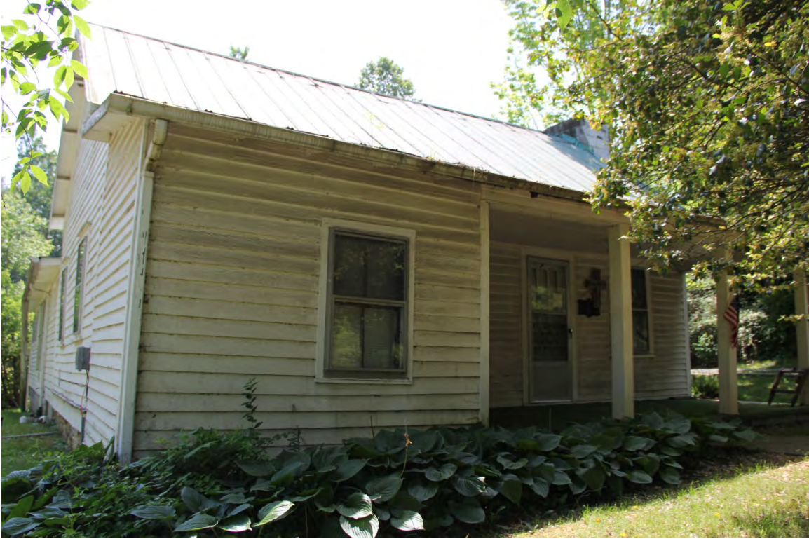
Mackey House, façade, view to southeast
