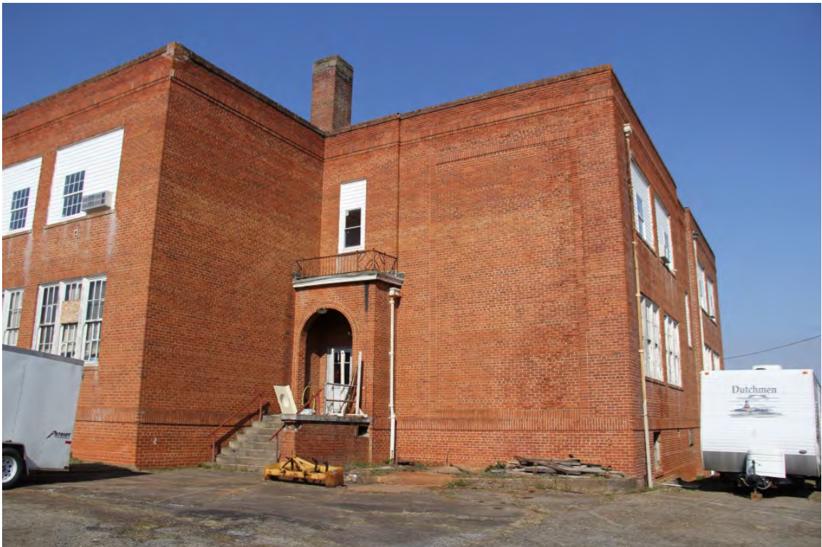
North wing, oblique view to west
