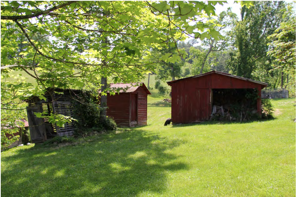
Outbuildings, view to southeast
