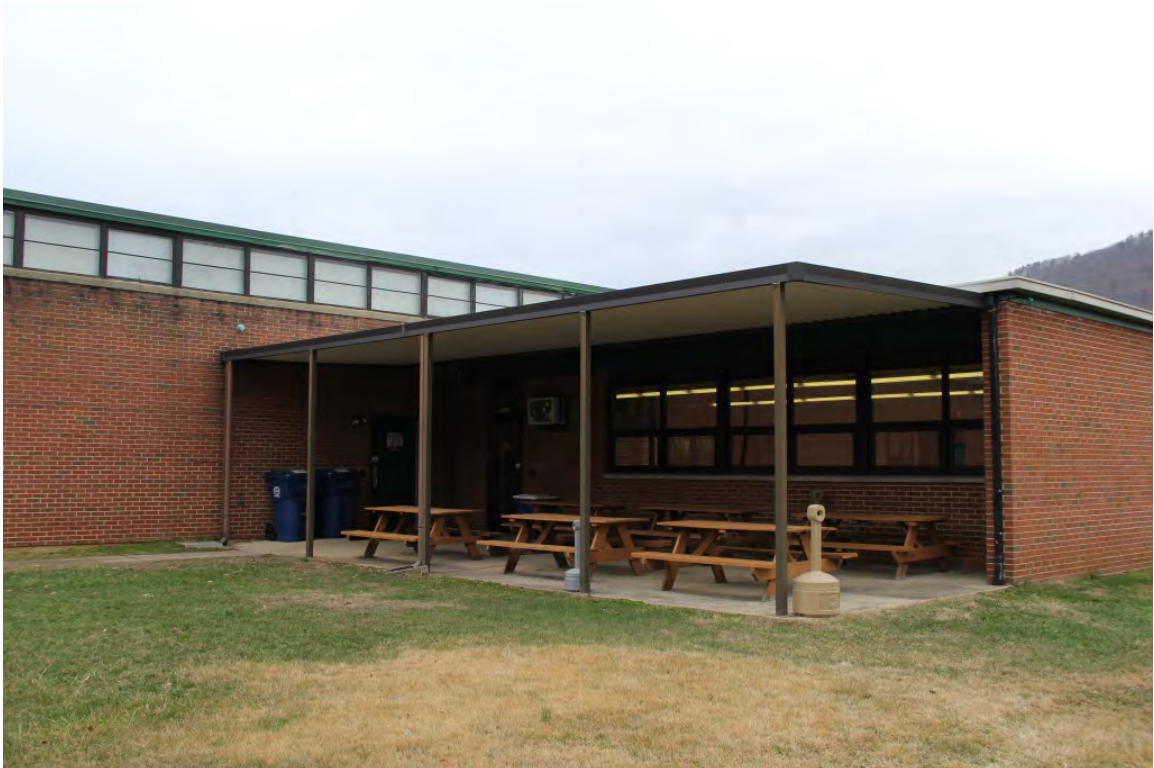
Mills Manufacturing, break room and patio, oblique view to northeast
