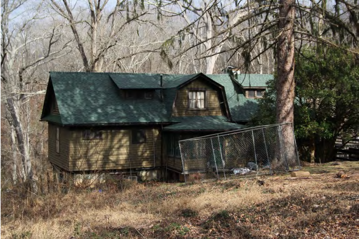
Glaser House, oblique front view to north
