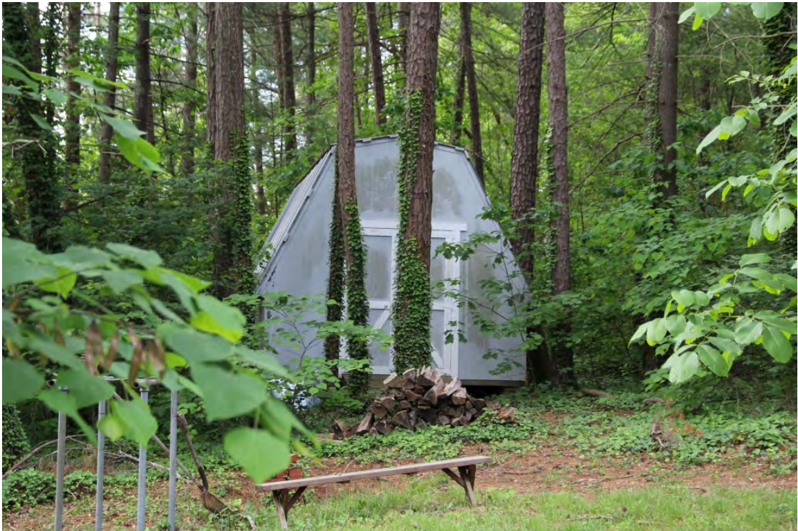
Storage building, view to southwest
