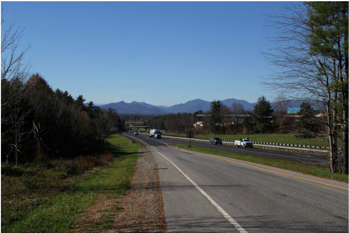
View southwest along US 19-23 from Exit 18, Monticello Road
