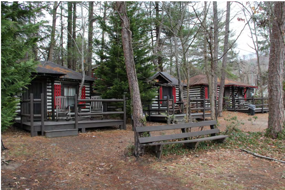
Cabin row, view to northeast
