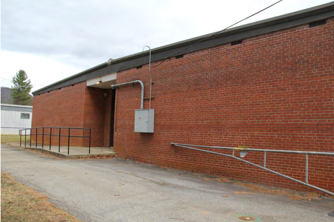
North classroom wing, north elevation, view to southeast
