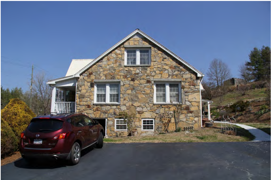
Banks House, south side elevation, view to north
