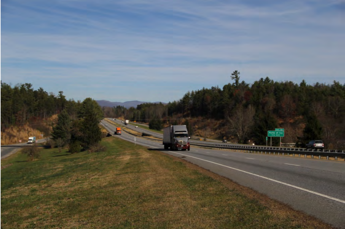
View north along US 19-23 at NC 197 (Barnardsville Highway) interchange, Exit 15
