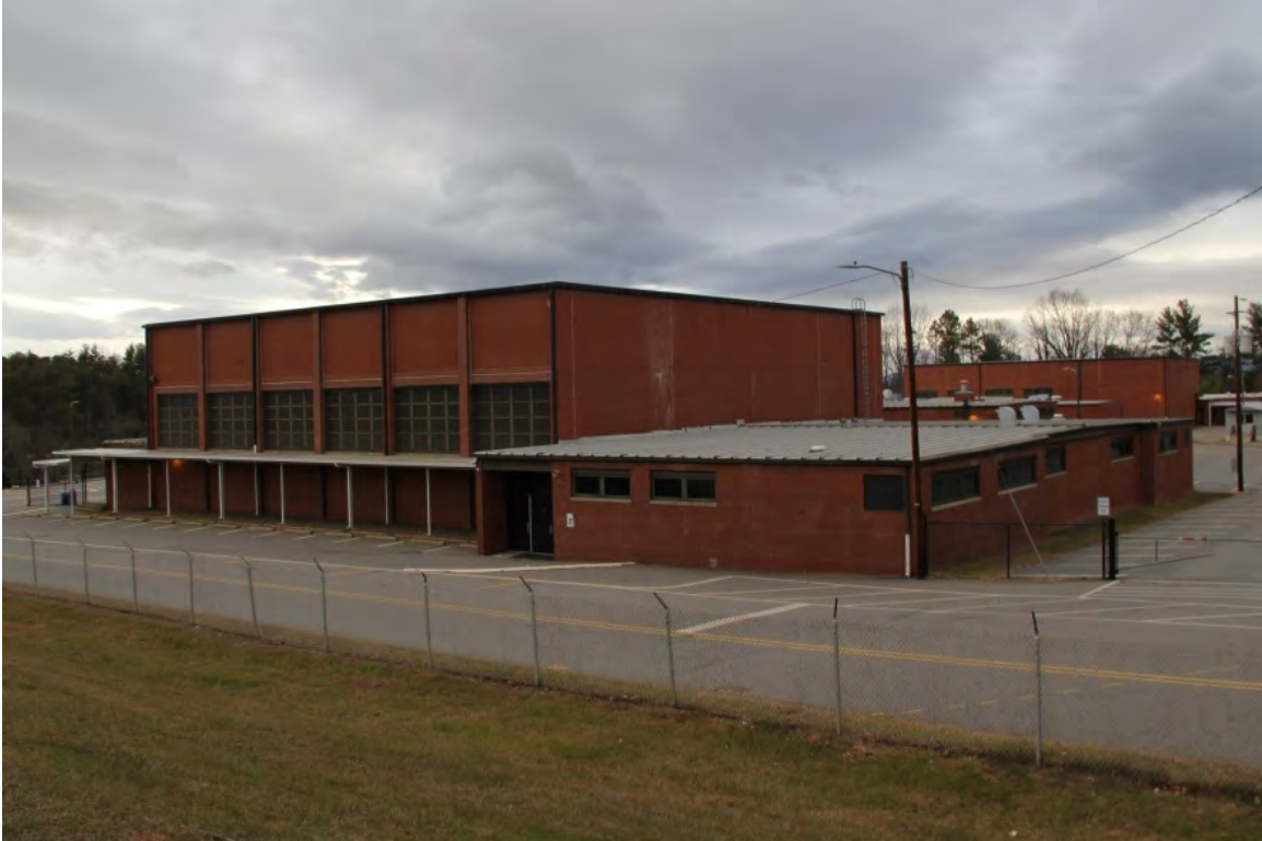
Gymnasium, oblique rear view to northwest
