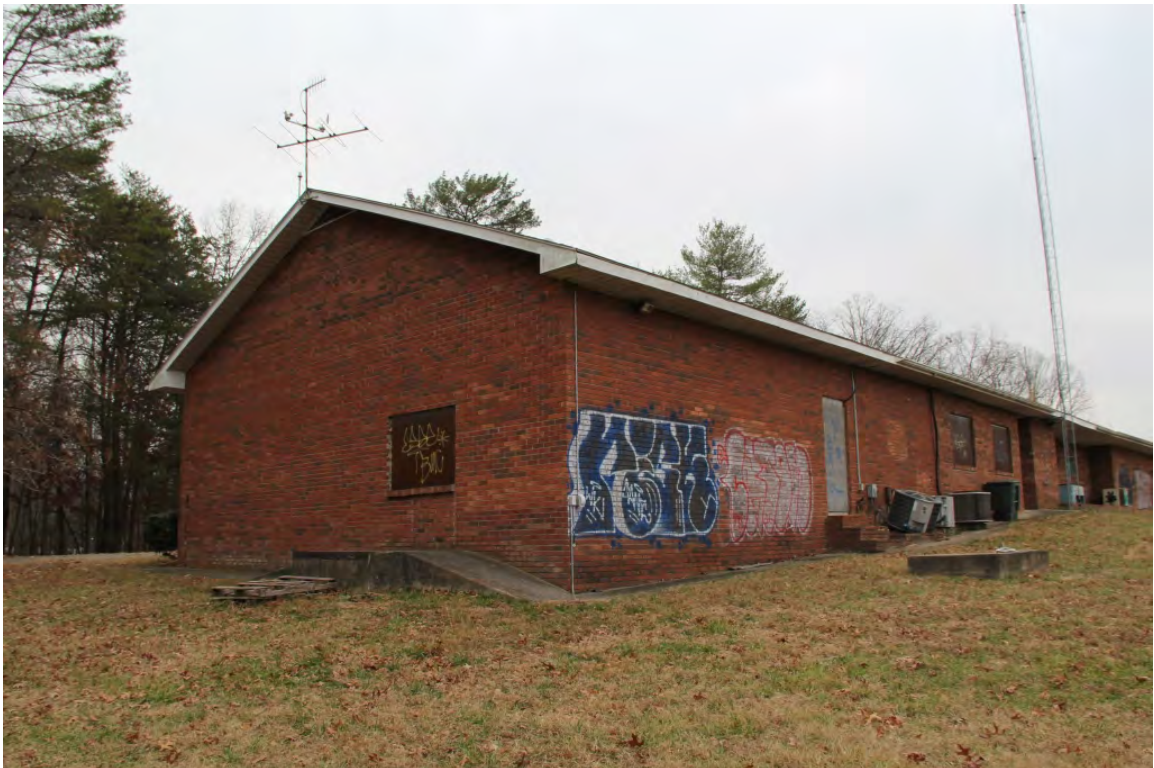
WISE Office, oblique rear view to southeast
