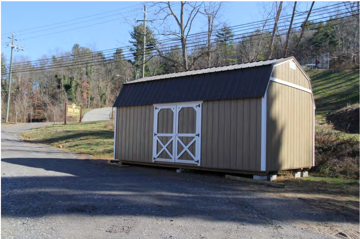
Storage building, ca. 2016, view to east
