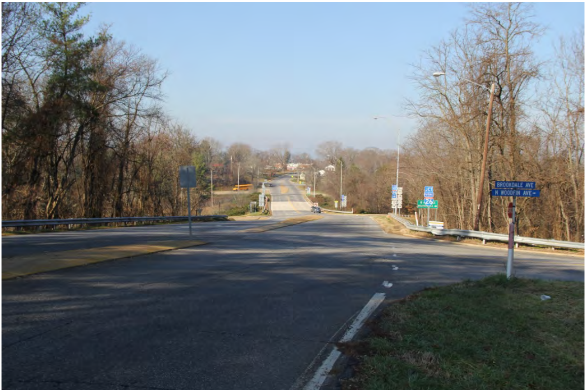
Elk Mountain Road over US 19-23 (Exit 24), view to west
