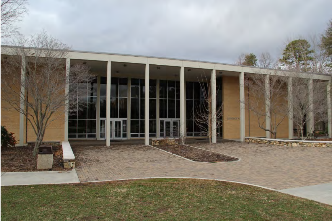
(#10) Lipinsky Hall (1964), façade, view to northwest
