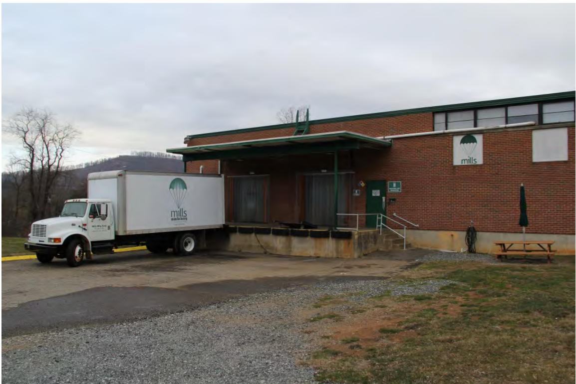
Mills Manufacturing, loading bays, oblique view to northeast
