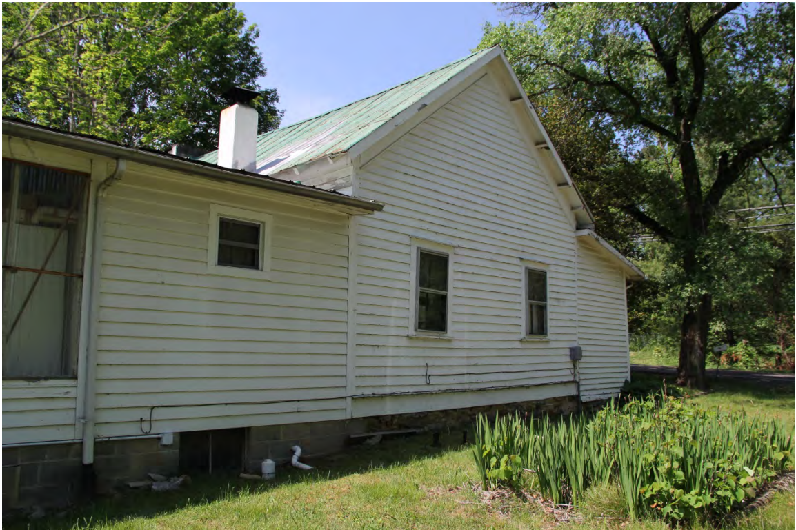
Mackey House, oblique rear view to southwest
