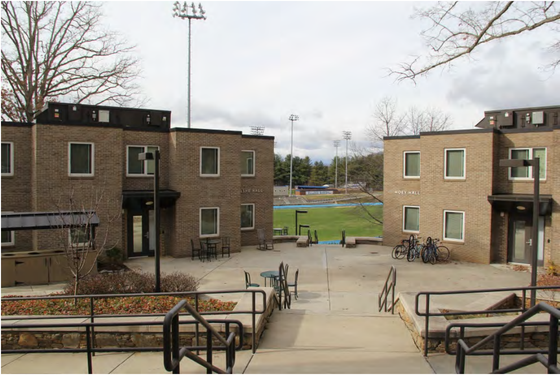
Governors Village Dormitories (1967) – (#25) Ashe Hall (l), and (#29) Hoey Hall (r), view to northwest
