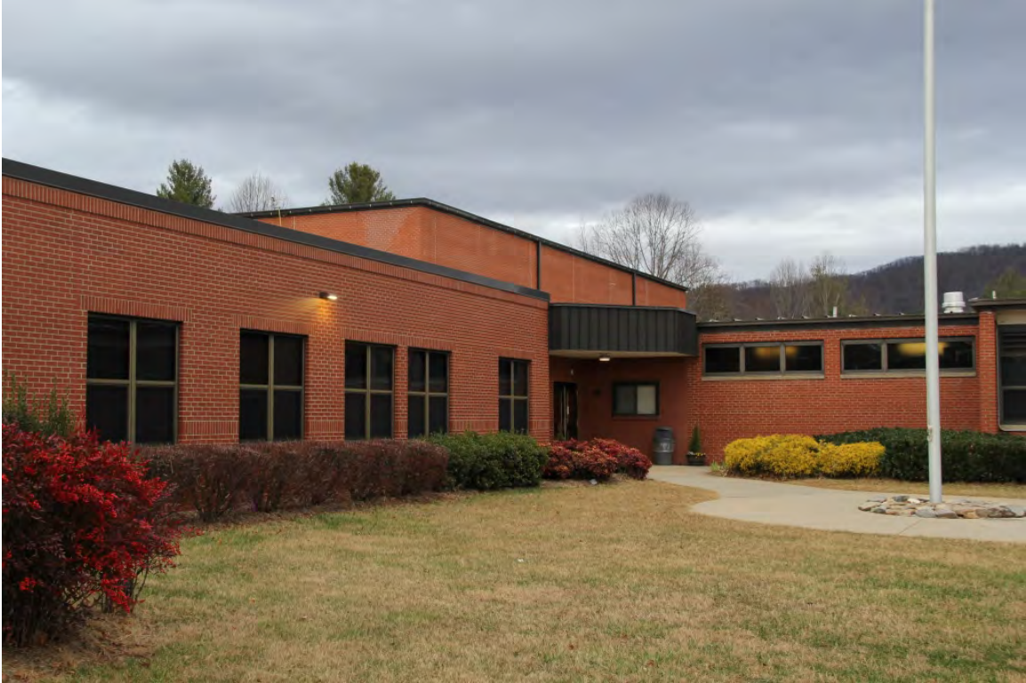
Administration wing (I) and main entrance, oblique view to north
