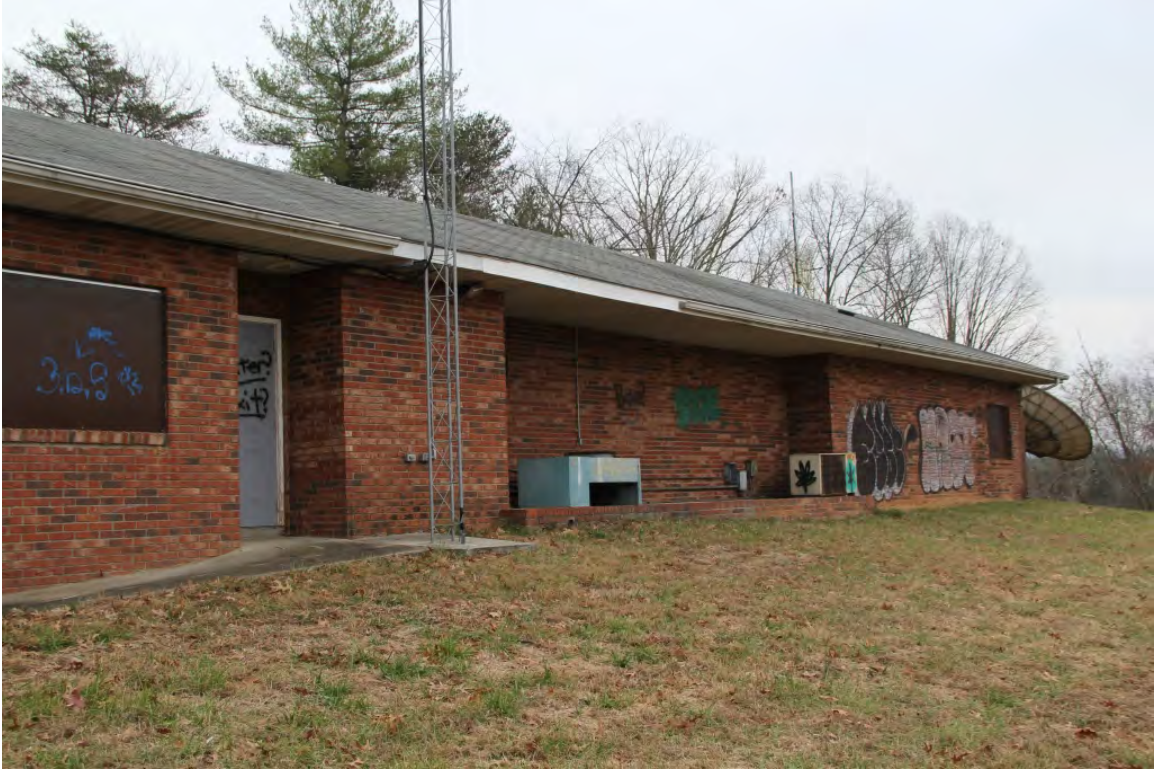
WISE Office, rear elevation, view to northwest
