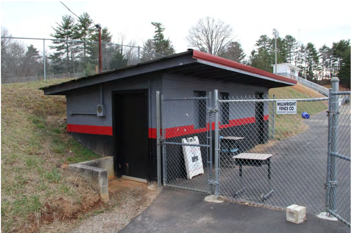
Ticket booth, oblique front view to south
