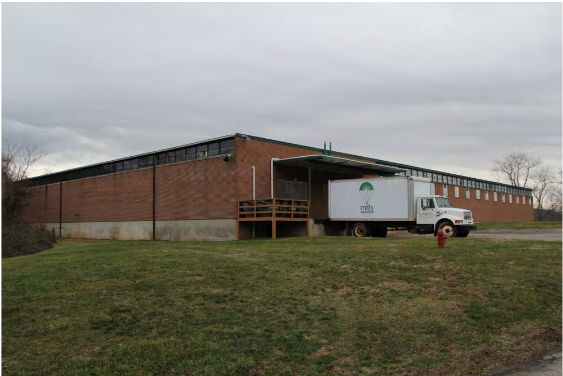
Mills Manufacturing, oblique view to southeast
